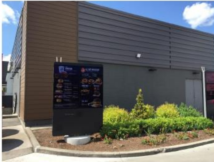
Installed signs at the Stone Rd W location.
